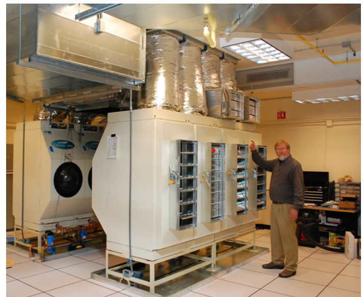
NSIDC technical services manager David Gallaher points out features of the new cooling units during the construction of the NSIDC Green Data Center. A key element of the redesign, these new evaporative units reduce cooling energy by more than 90 percent, compared to the traditional air conditioning units that they replaced. (Credit: Ron Weaver, NSIDC)
